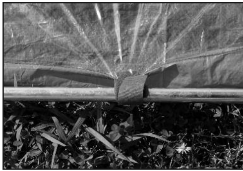
STEP 4 - Secure shelter skin by attaching the velcro to the frame.
