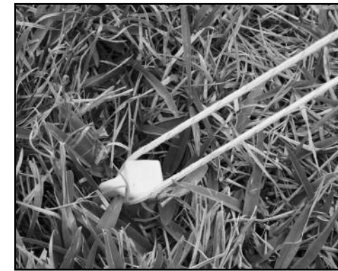
STEP 15 - Loop this around the stake's head and push into the ground.
