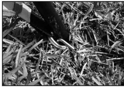
STEP 11 - Stake down at all pin and rings.
